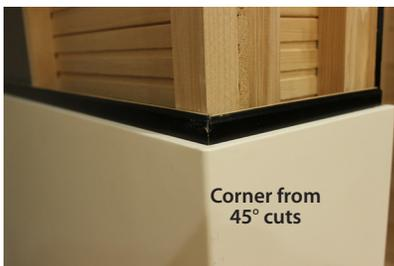
Position pieces of trim behind the lip of the exterior panels so that the 45-degree cuts are meeting each other at the corner of the sauna. (Image 50) Continue assembly of exterior panels.
