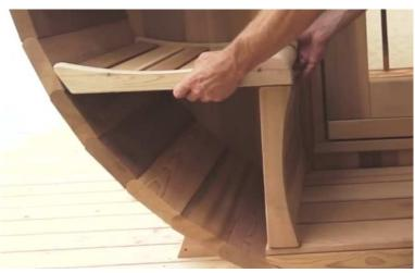
Flat Floor option: (included with Signature Contoured Benches option) Place the fully assembled flat floor in the sauna, and make sure it is level.
