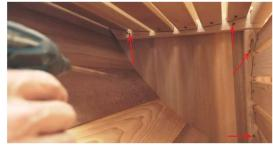
Also fasten from the outside through the outer wall into the back of the bench seat frame with 2 %" screws (1 place).
