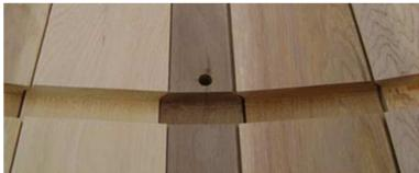
A half-inch hole was bored for drainage just inside the walls on the lower special stave.
