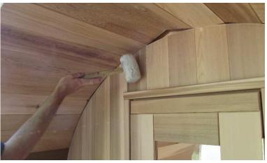
This is how the sauna normally looks at this stage. The barrel will be adjusted later with a rubber mallet to eliminate this hump.
