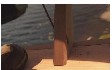
To fasten the curved bench in the dome, first attach a support bracket to the dome-end of both benches with three 2½" deck screws each.
