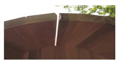
all the way to the line. The line is just a guide to keep the round shape. Leave as much of a gap as possible. This will make it easier to fit in the last staves at the top and shape the barrel.
