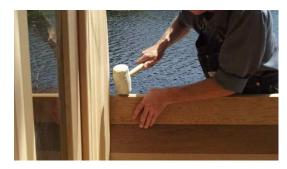
Again, make sure the inside faces of the staves follow with the pencil circle on the end walls to get a nice round circlular shape to the barrel.
