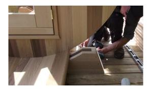
Position the temporary stave-holder stands on either side of the dome approximately 1½" away from the edge of the dome. You can use screws or spikes to hold them in place.
