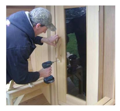
The door handle usually goes in the centre of the door (left) and the Towel Bar is made to go on the inside of the door (below) but can be installed lower or higher as desired. It usually goes about half-way vertically. Use 1½"screws.
