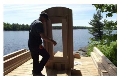
Place the middle section of the front wall with the door into the groove in the staves.
