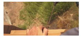
Lay down the curved dome bench and fasten it to the support brackets with 2½" deck screws. (2 places per side)
