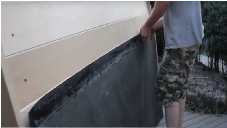
31. Starting flush to bottom of sauna, apply shield with the top side adhesive edge oriented upward.
