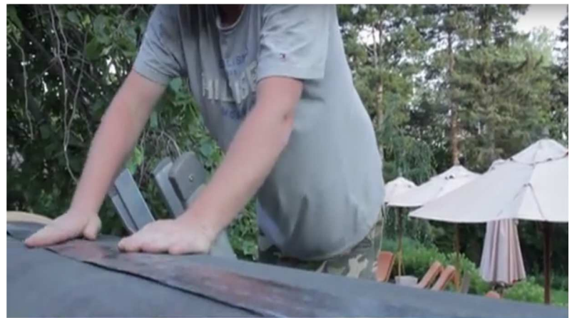
34. Overlap the shield at top for a good seal.
