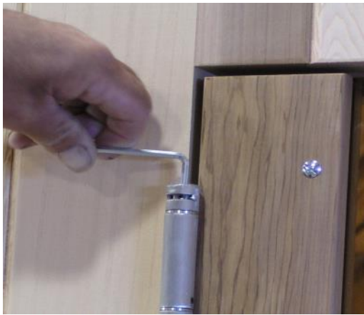
Adjust tension with hex wrench
