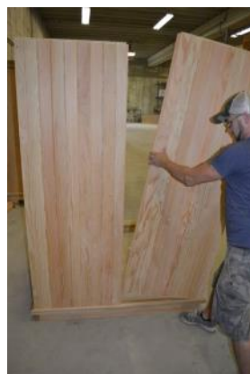
Position Wall Section I
