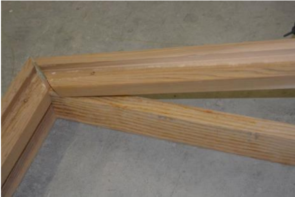
Position wall support rails
