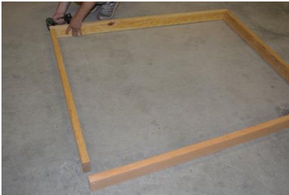
Assemble floor riser
