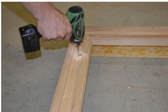
Fasten wall support rails to floor riser
