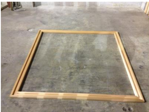
Completed Roof Support
