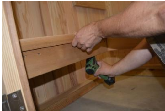
Attach Foot Rest and Lower Side Bench
