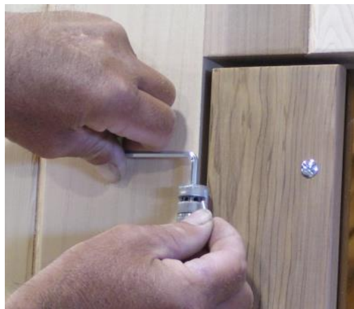
Insert pin and relax tension to hold
