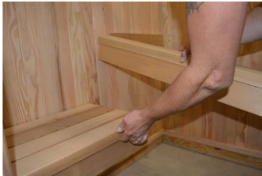
Attach Foot Rest and Lower Side Bench
