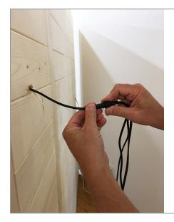
**STEP 5** - On the exterior of the sauna connect the power supply to the LED bar cord. NOTE: Be sure the connection is secure and the nut is firmly hand-tightened.
