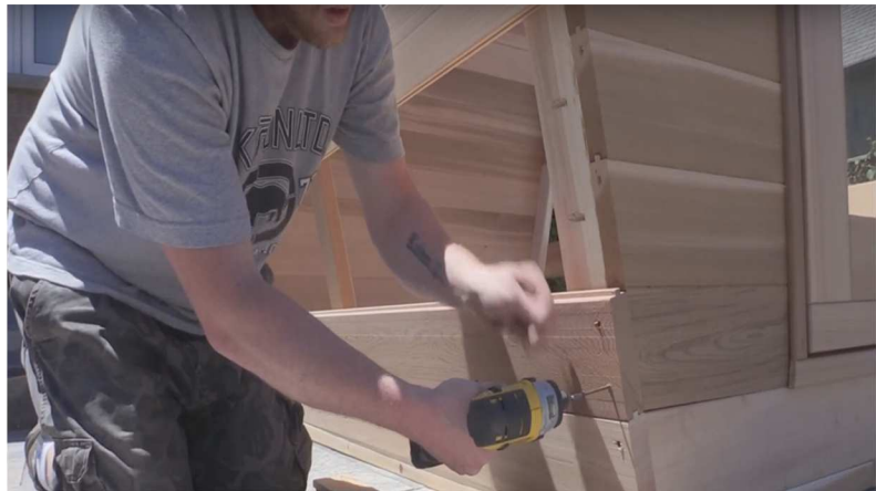
24. Continue to build wall upwards securing screws into staves at ends and middle support as stated before.
