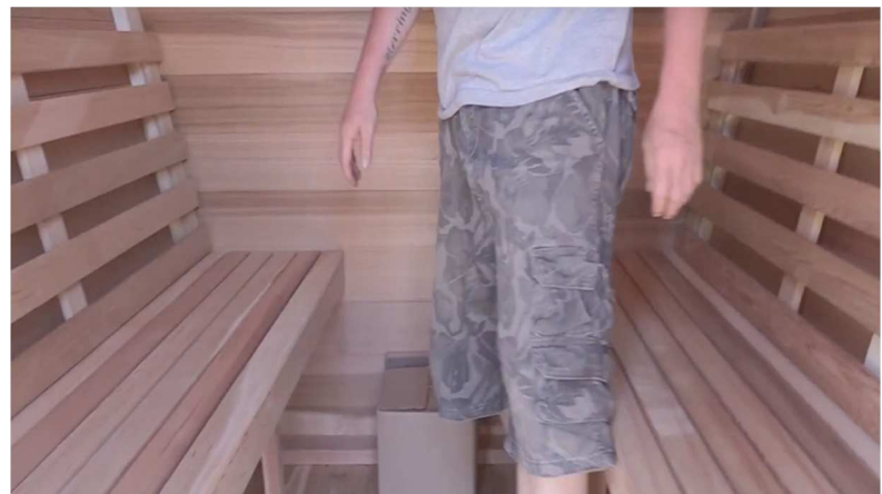
60. Place the heater on top of the "box of rocks" to install at the correct height.
