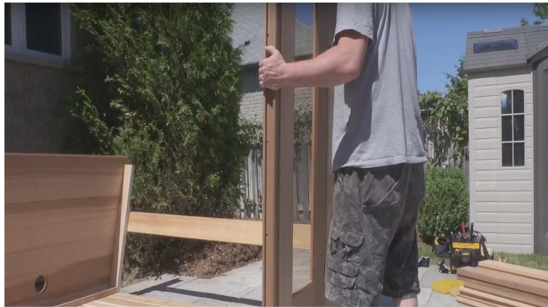
10. Slide door into place on the front wall.
