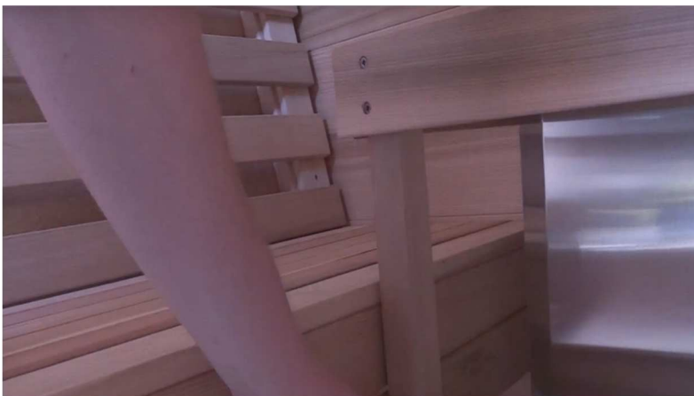
69. Make sure the center of the heater guard is at same level as the top of the bench.
