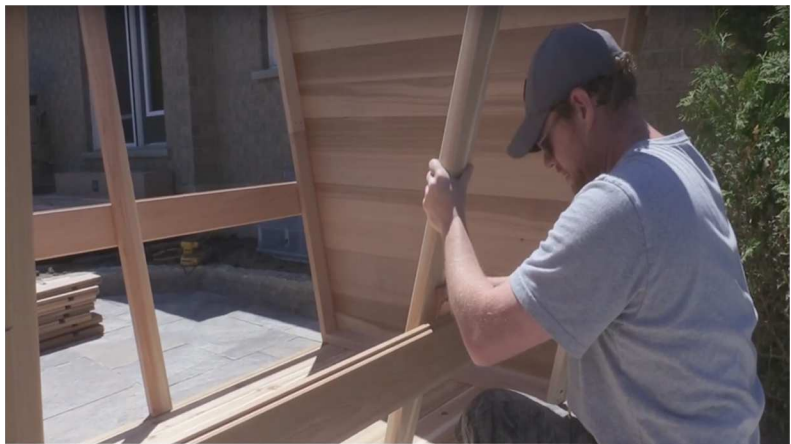
18. Using 2 1/2" screws, attach middle support in center of sauna. Make sure support is flush to edge.
