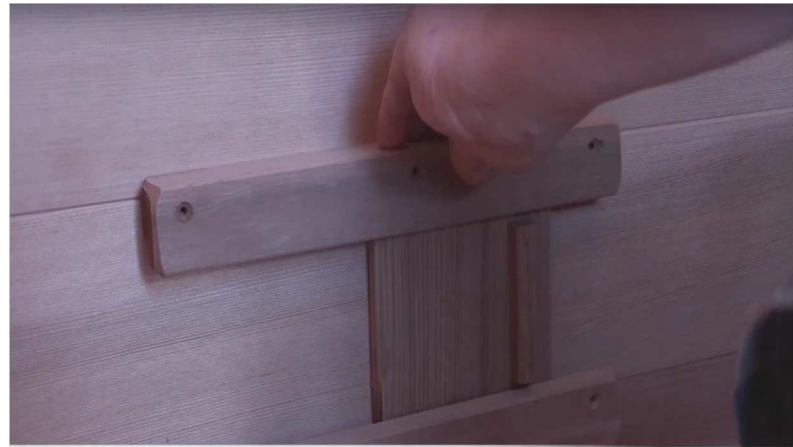
50. Make sure when securing the top vent cover rail that the vent cover can still move with ease. Be careful not to overtighten.
