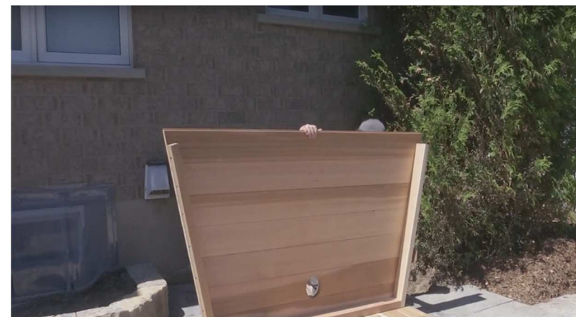
6. Using 2 1/2" screws, screw back bottom piece into floor.
