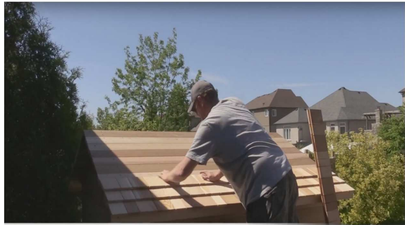
38. Continue attaching shakes, working up to peak on either side.
