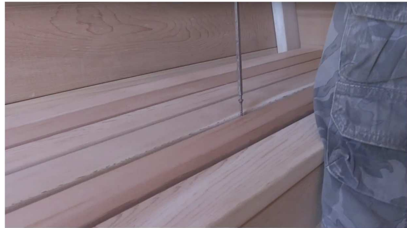
56. With 2" screws, screw bench down to supports through spaces in bench.
