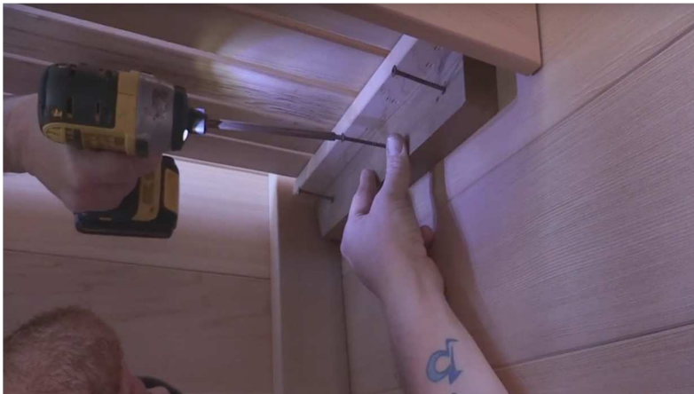
57. The seat supports should sit under the pre attached bench supports.
