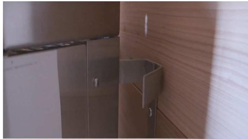
64. Place heater on wall brackets.
