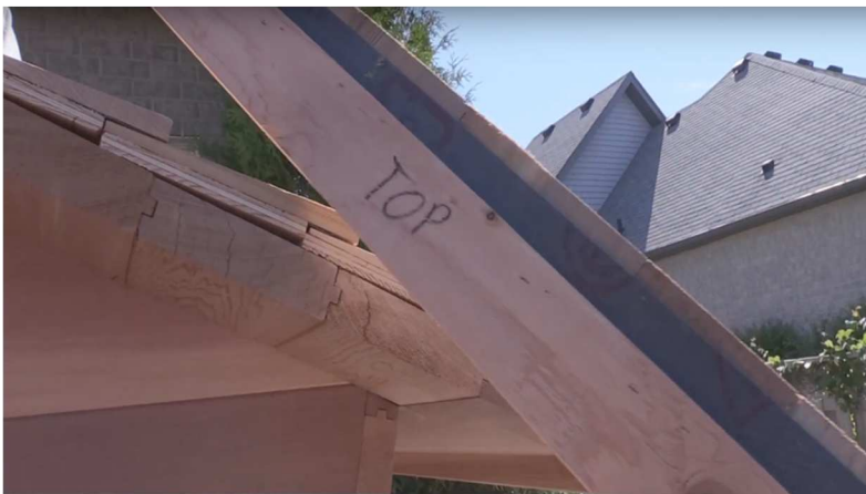
39. Attach piece marked "top" at peak of roof.
