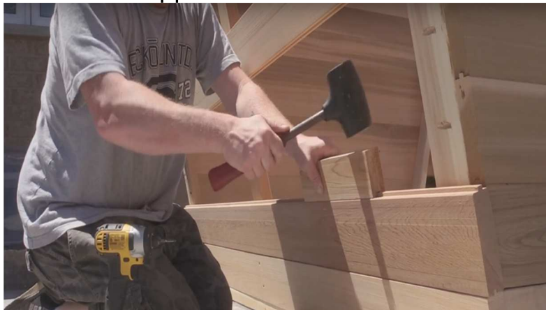
23. Use provided block to "tap" wall staves into each other. Failing to use block could result in damage to "tongue" of stave.
