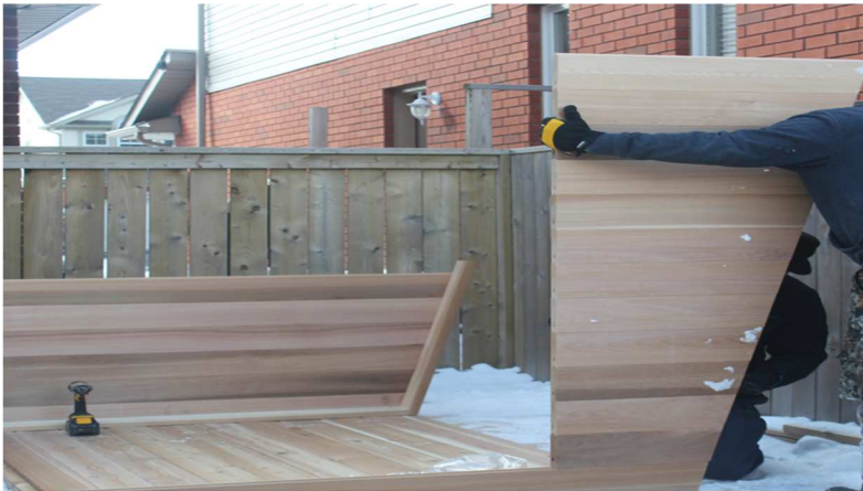
7. Attach front side wall onto front bottom.
