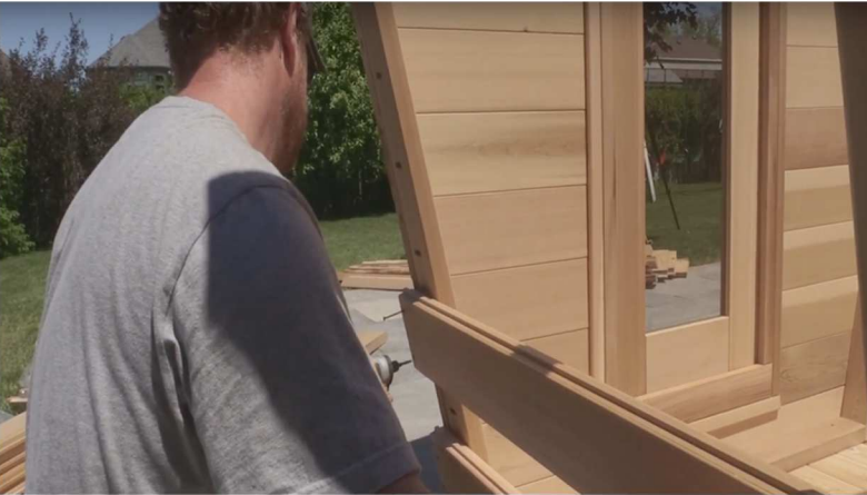
25. Lower the previous "support stave" to fit with the other staves.
