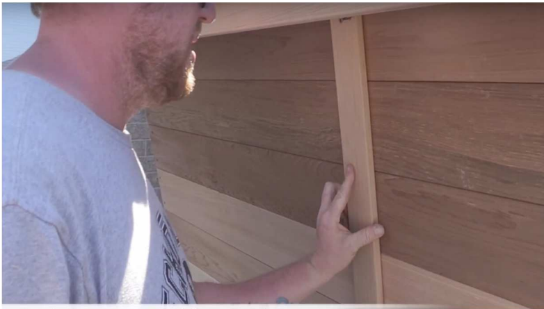
43. Attach trim pieces using 1 1/2" screws in the pre drilled holes on front and side corners.
