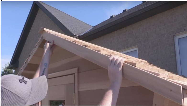
45. Attach roof trim using 1 1/2" screws.
