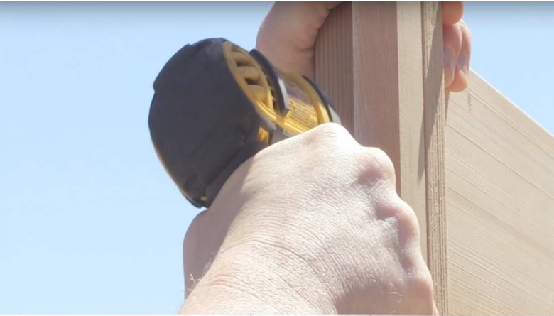
13. Fasten other side of door 2-3" from top and bottom and in center through door trim using 2 1/2" screws.
