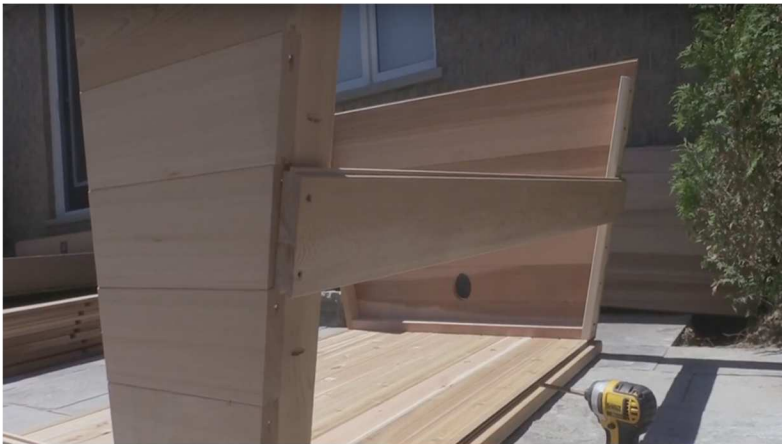
9. Square up front and back walls and screw a wall stave into front and back walls for support.
