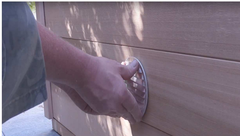
47. Place vent inside hole on back wall from the outside while keeping it level.
