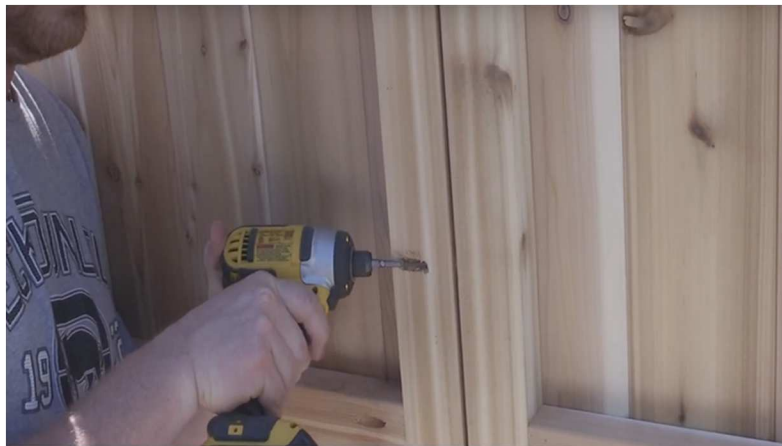
3. Screw floor pieces together in pre drilled holes using provided 2 1/2" screws.
