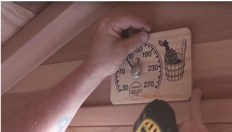
51. Install the thermometer centered above the door using a 1 1/2" screw.
