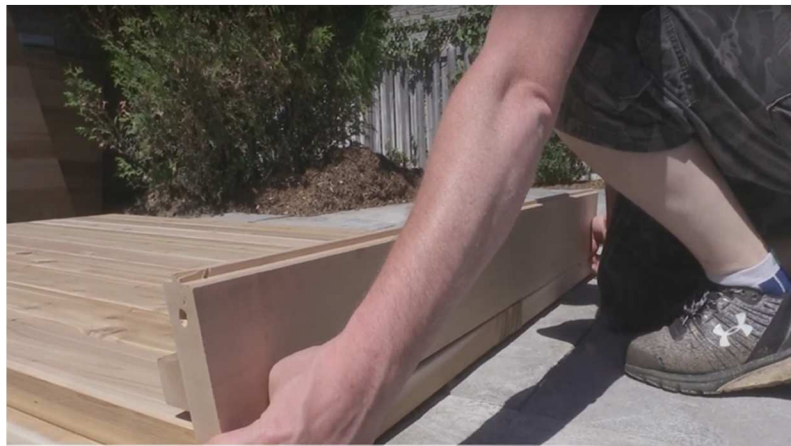
4. Place front bottom so it is flush on either end.
