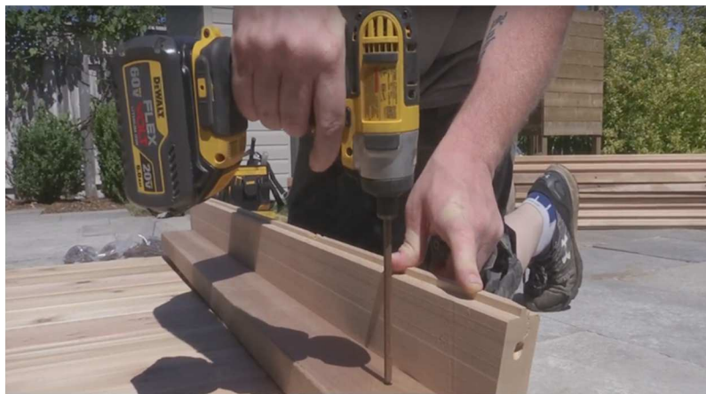
5. Using 2 1/2" screws, screw front bottom into floor in pre drilled holes.
