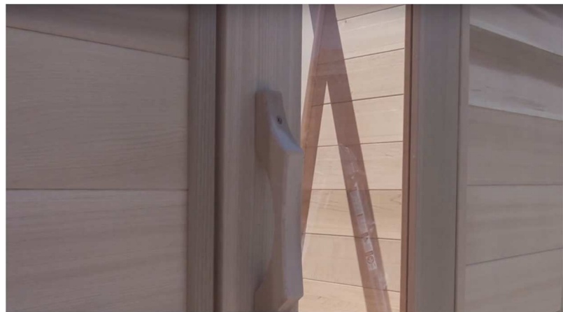
42. Install the door handle outside at desired height with 2" screws.
