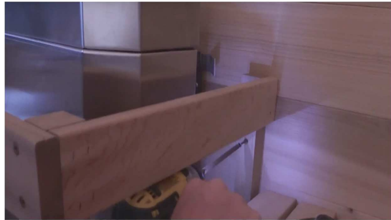
68. Attach heater guard to wall with 2" screws using pre drilled holes.
