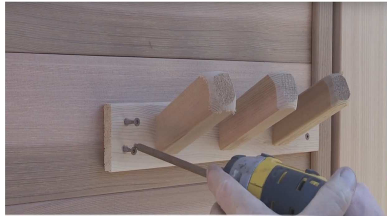
46. Using 2" screws, attach towel hanger at desired height outside the door.
