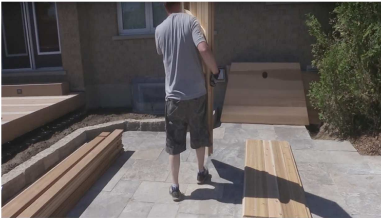
1. Start by placing both floor pieces on level ground.
