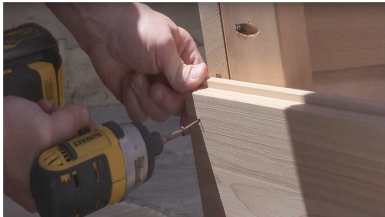
22. Keep screws in 1" from edge to ensure they will be covered by trim.
