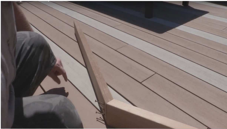
19. Screw top support pieces together using 2 1/2" screws.
