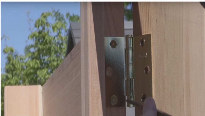
11. Ensure door is square and fasten hinges using 2 1/2" screws.
