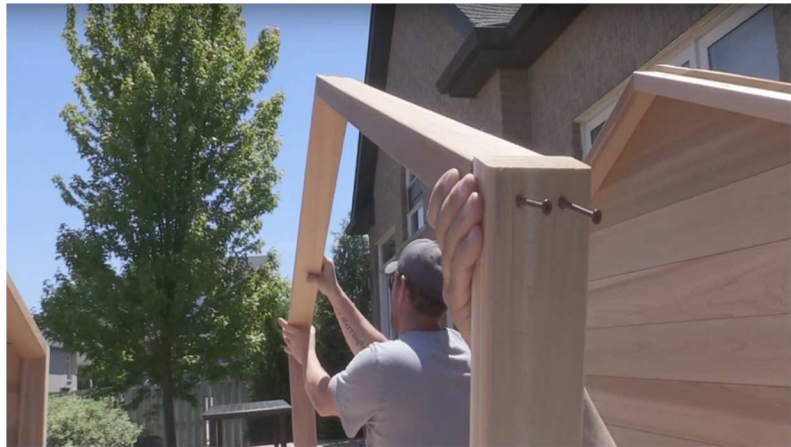
20. Screw top support pieces into middle supports using 2 1/2" screws.
