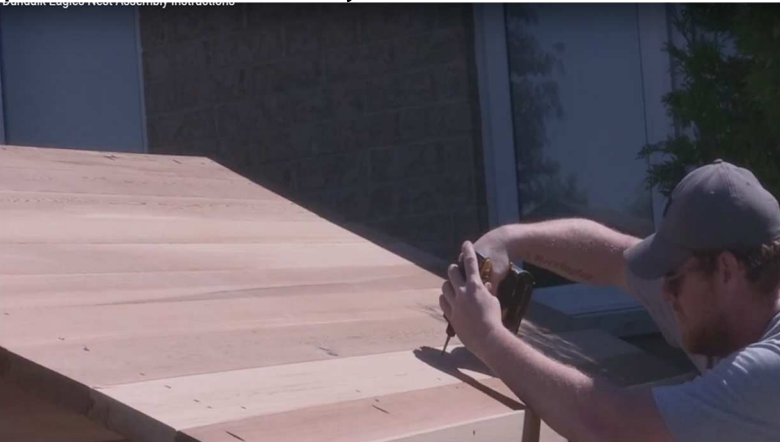
35. Use (6) - 2 1/2" screws per staff. (2 at each end and 2 into center support)
