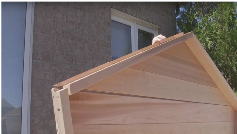
17. Attach top back, using same steps as front top.
