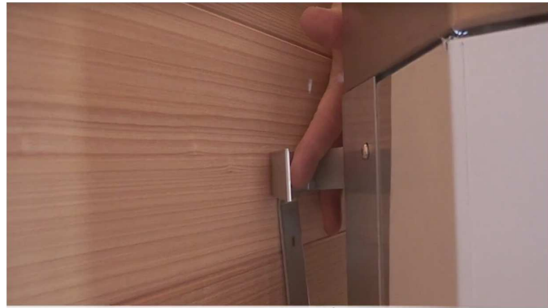
62. Mark the wall placement of the heater brackets.
