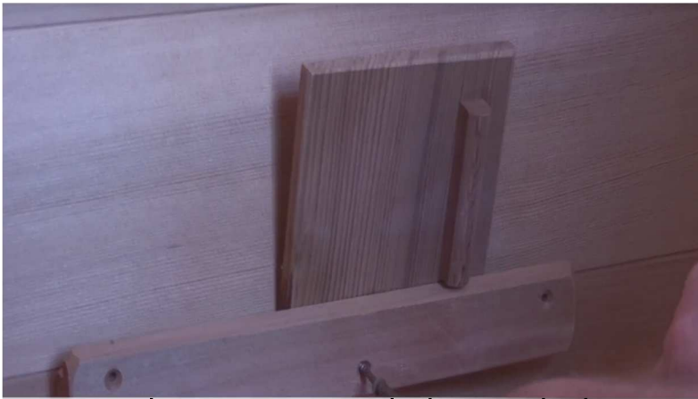
49. Using the cover as a guide, line up the lower rail and secure with 1 1/2" screws.
