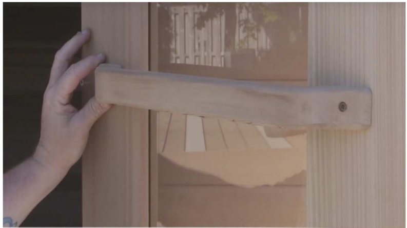
52. Install towel bar cross-ways on inside of door at desired height using 2" screws.
