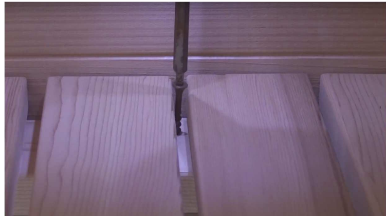
58. With 2" screws, screw bench down to supports through the spaces in bench.
