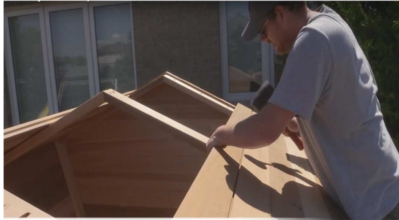
32. Continue adding roof staves working your way up the roof on either side. Do not screw in roof staves at this time!
