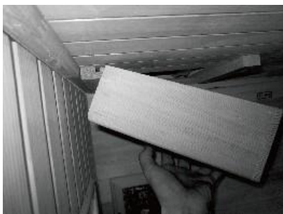
FIG 15.2 Installing the Radio Wood Housing
