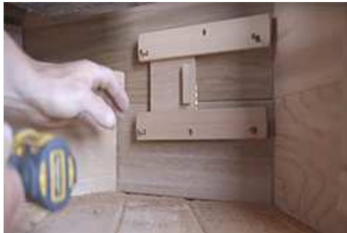
Ensure the vent cover slides freely before screwing in tightly
