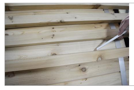
**STEP 2** - Center one of the roof sections over the radius of the barrel with the center slat directly above the door of the sauna. Make a mark above the last slat on each side and remove the roof section.
