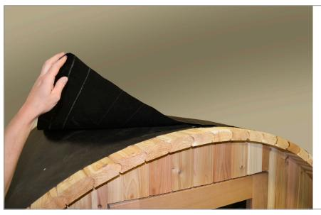
**STEP 4** - Center the third piece of felt over the two side pieces and secure with (2) roofing nails so that it stays in place.
