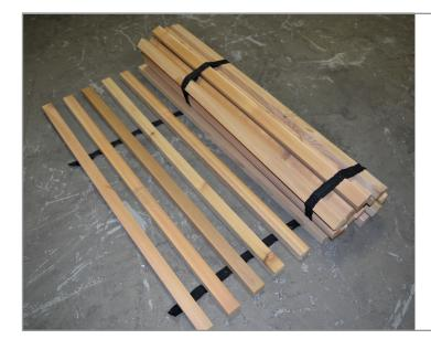
**STEP 1** - Roll out the roof sections so that the black straps connecting the slats is facing down. Find the center slat.
