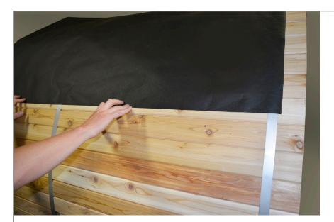
STEP 3 - Line up the edge of one of the felt roof pieces and be sure it runs parallel to the stave boards. It must cover the band on each side before nailing in place with (2) roofing nails. Do this on both sides of the sauna. (Note: The roofing nails are only intended to hold the felt in place for now. It is the roof sections that will actually secure the felt in place.)
