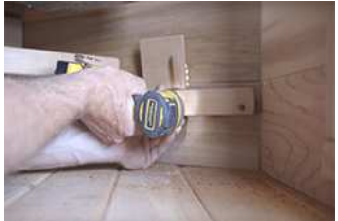
Secure the vent cover pieces with 1 ½" screws as shown.
