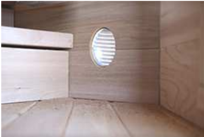
Using supplied screws, secure vent on the inside of sauna.
